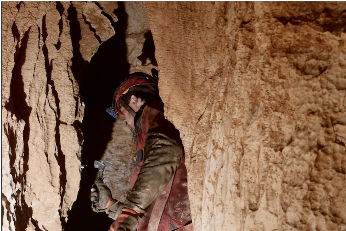
Figure 110: Jack hammers the M8, stainless steel raul bolt we use on expedition to secure a traverse line over MIGHTY FINE INDEED 3rd Pitch, a respectable P42, before drilling in a signature Y-hang: an airy take-off over a diminishing ledge which provides a beautifully clean hang 📷 Tanguy Racine
