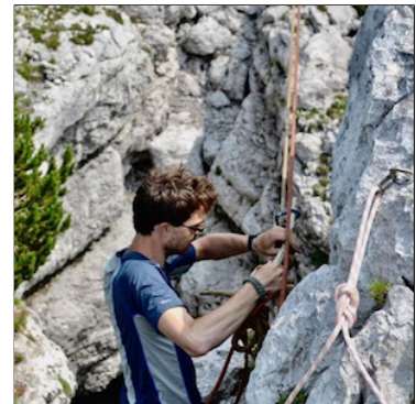
Figure 70: Jack Hare sets up the hauling system and we find an elegant solution to specifically send the pulley out over the pitch and retrieve it 📷 Rhys Tyers
